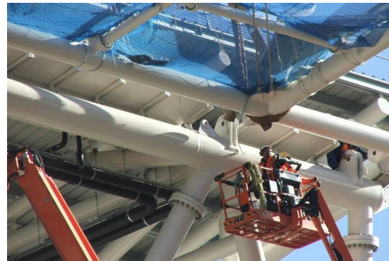
Figure 9: Safety net installation using a mobile elevating work platform.
